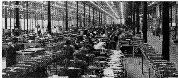
The Scarmagno factory.
